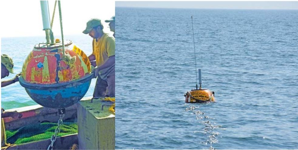
Photograph showing wave rider buoy installation
